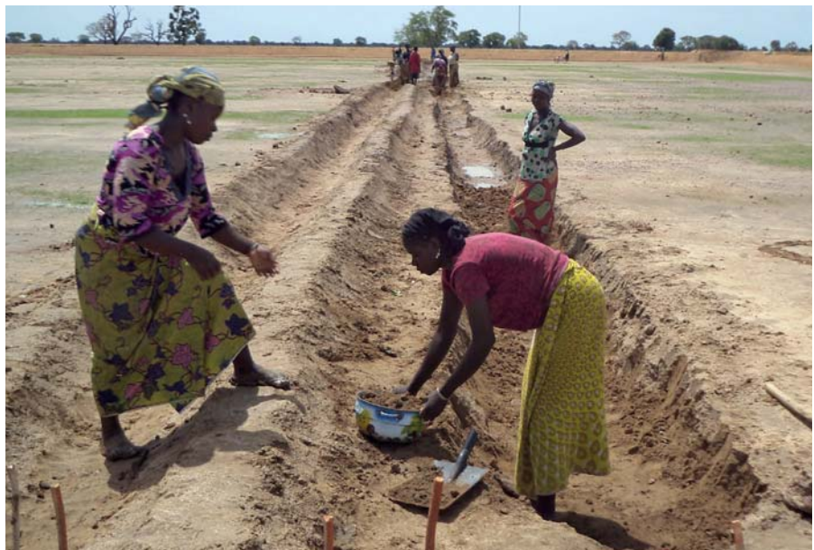
Women from the project helping to build the quaternary canal for their lots.
