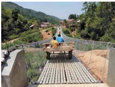
The tractorable Skan bridge in Laos.
