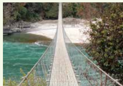
A pedestrian suspended bridge in Nepal.
