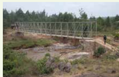
A pedestrian truss bridge in Nepal.
