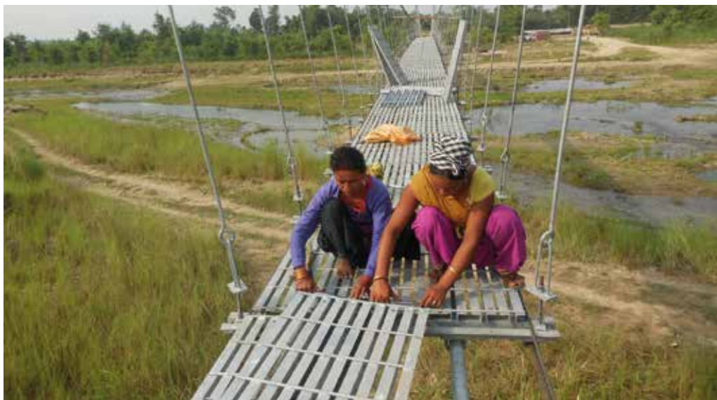
Women fitting a steel deck on Ghurswaghat Bridge, Kanchanpur.
